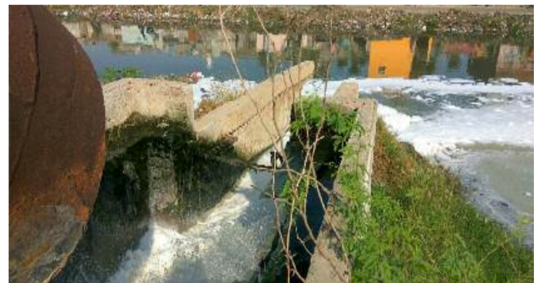
Effluents being let into the Buckingham Canal at Neelankarai | SHILAJIT M
