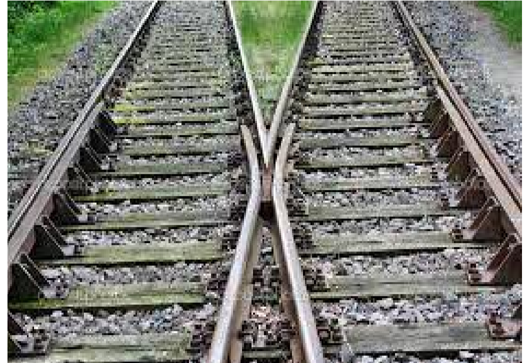
Joints are where cracks are most likely to develop | DEPOSITPHOTOS
