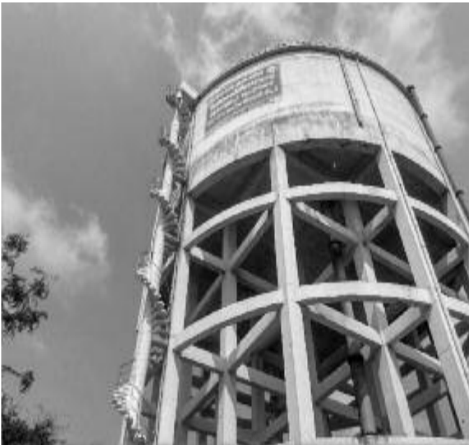
Water tank at Thiruvottiyur | U.M. ABHIJITH
