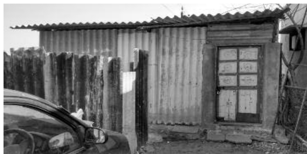
Encroached area near Pallikaranai Marsh.
