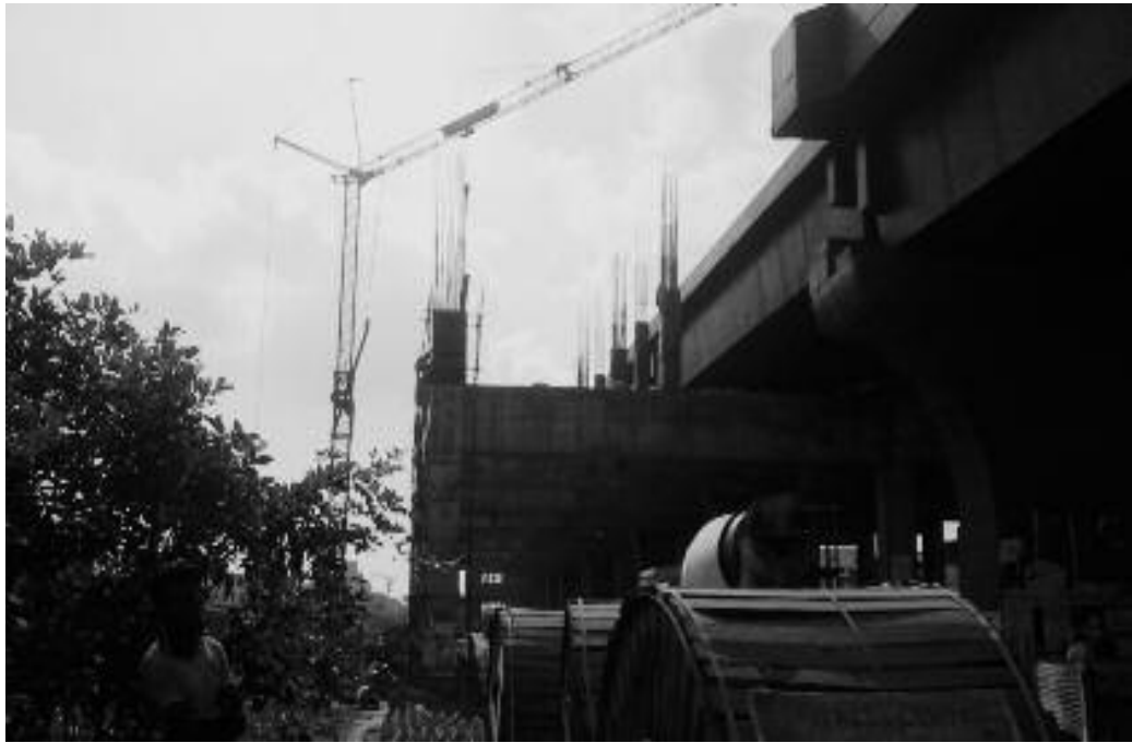
Work in progress at the Puzhuthivakkam MRTS station
