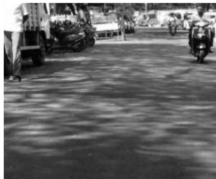
Pycrofts Garden road in Nungambakkam was relaid recently.
